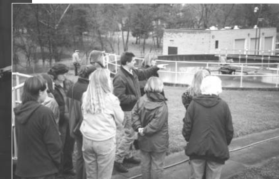
(Center) Tour leader Gordon Cruickshanks points to a circular secondary clarifying tank, a final step in the water clarifying process. (Right) Gordon Cruickshanks shows Water Strider student, John Tabor, a polymer tank. The chemical polymer is used to aid the clarification process at Waynesboro's Water Treatment Plant.
