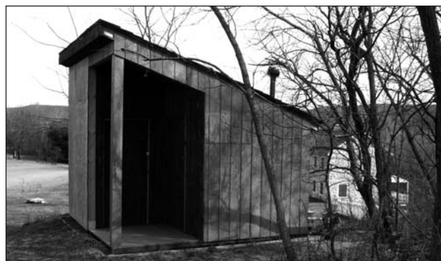
The composting toilets are housed in a historically appropriate new building constructed specifically for that purpose.
