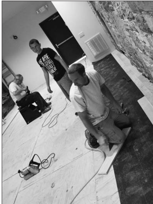
Lowe’s Heroes workers, left to right, Paul Mayes, Jeff Poffenberger & Jeremy Mays helped to expertly install wormy red oak floorboards in the converted wagon shed room. Photo by Tracy Holliday.
